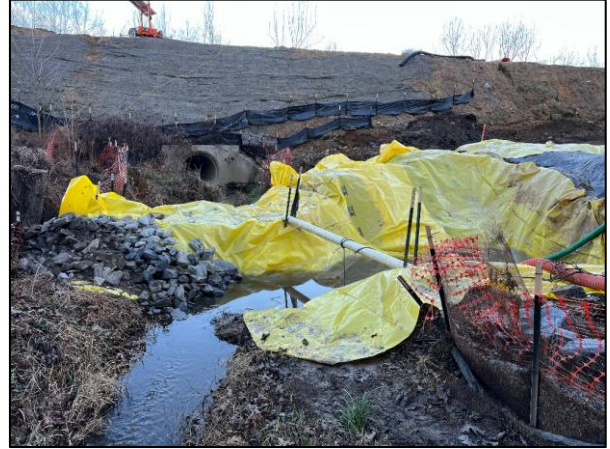
Construction stream diversion (lower Reach 4)
