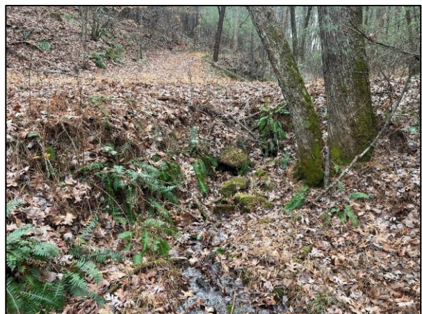
Photo Point 6 (UTFBR culvert facing upstream)
