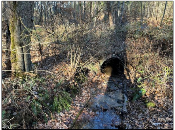
Photo Point 22 (UTFBR culvert, facing downstream)
