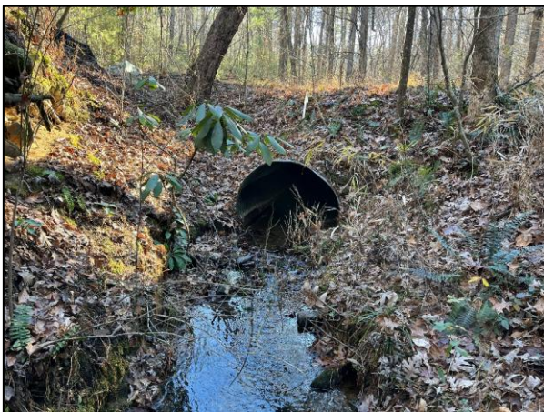
Photo Point 23 (UTFBR culvert, facing upstream)
